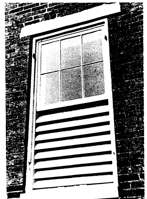
Figure 3. The exposed edges of the louver slats were plumb cut in order to create a water drip on the exterior. For aesthetic reasons, the louvers were painted the same color as the sash and trim. Photo: Charles Fisher
