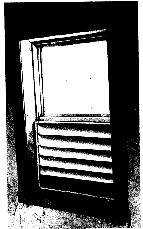
Figure 5. Screening was attached to the back side of the louvers to prevent the recurrence of insect, bird, and rodent infestation. Photo: Charles Fisher
