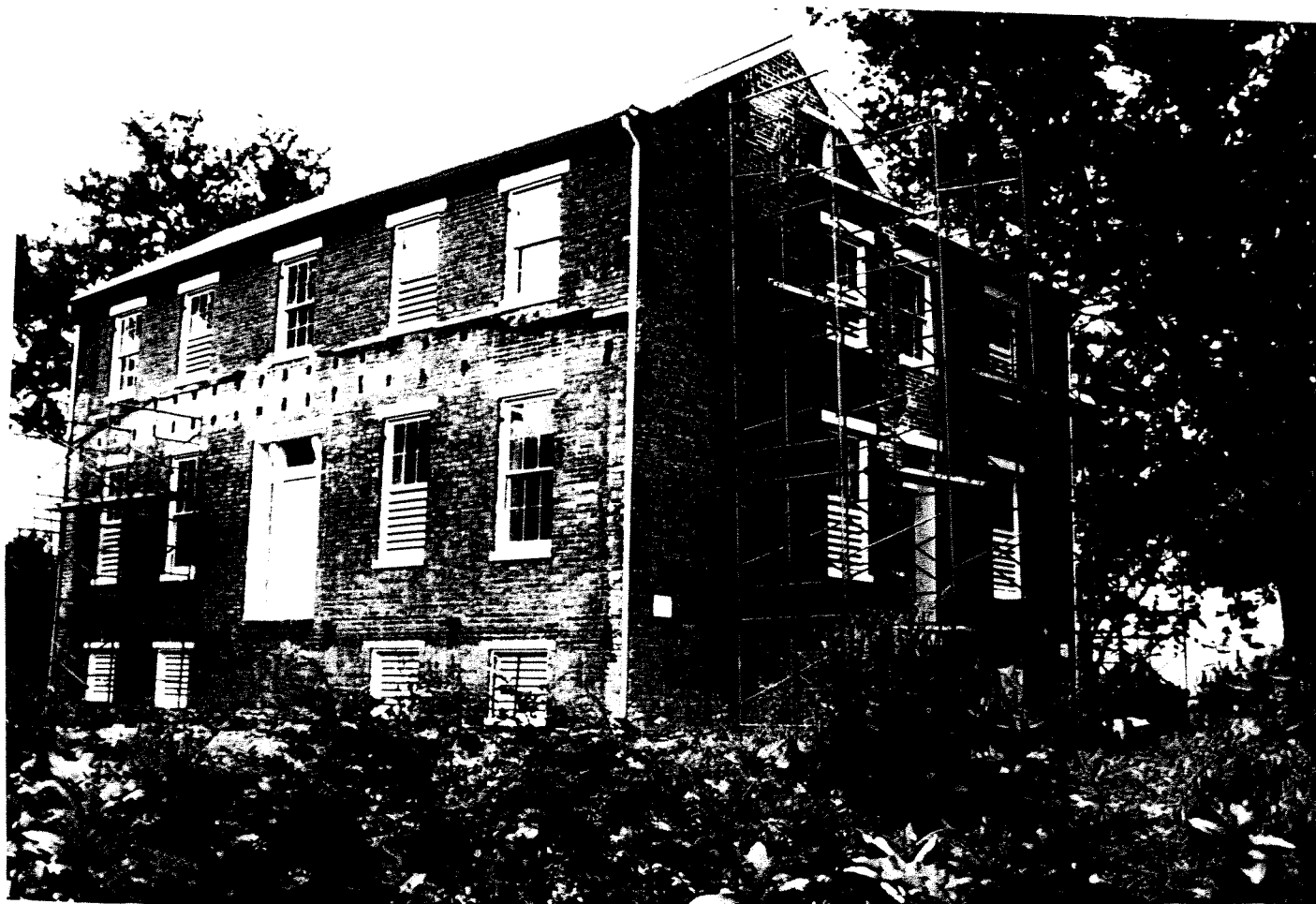
Figure 6. The window louvers installed in the Worthington House have proven effective over the past two years in providing the necessary ventilation for the building. Photo: Tom Vitanza.
